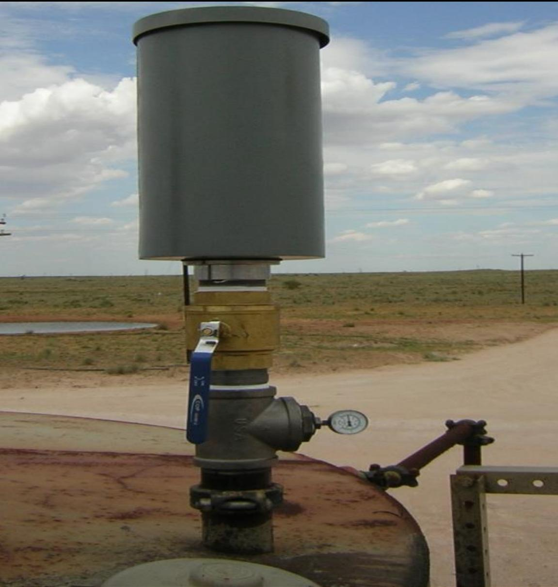
The Bio-Filter works on the absorption principle using a dry, glycol based media.
